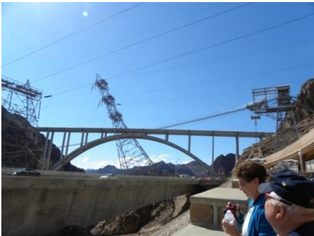
The new Bridge
